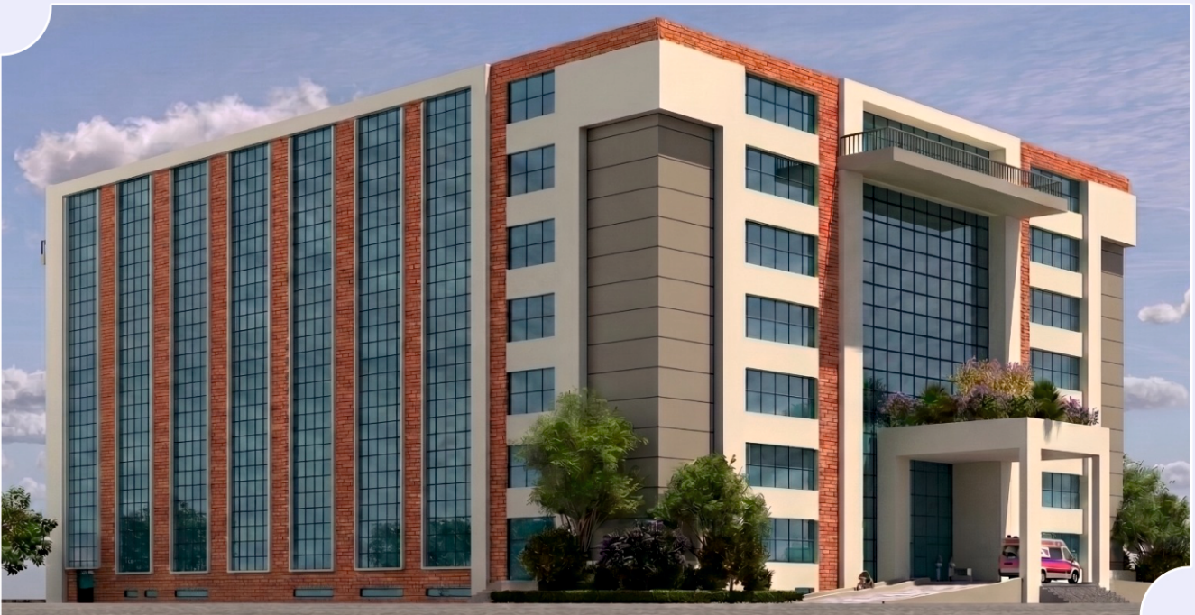
PGIMER CRITICAL CARE BLOCK Project Under Way
