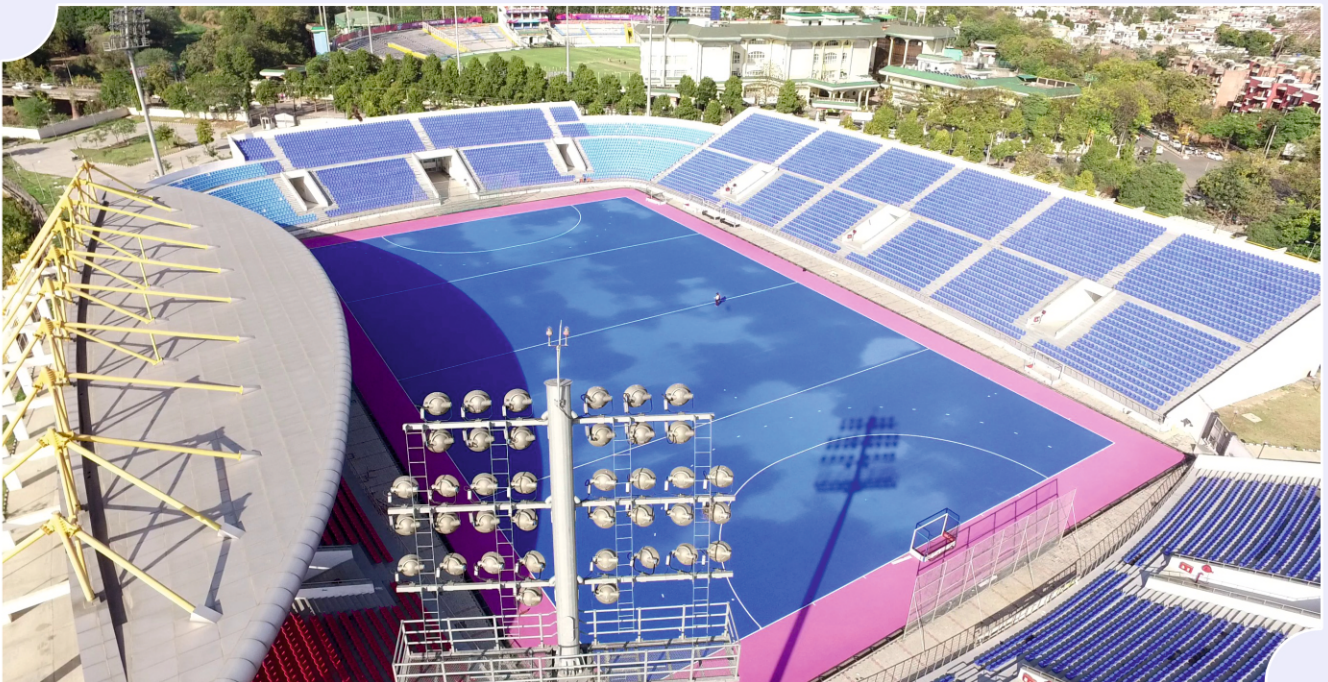
INTERNATIONAL HOCKEY STADIUM, MOHALI
